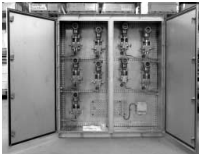
Heater plate mounted in a instrument enclosure.
